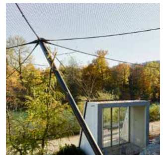
Image 8: Similar impression created by a fine-meshed Webnet of Jakob Rope Systems installed in a Zoo enclosure.
