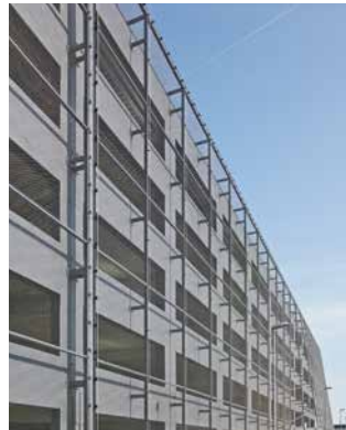
Image 12: Similar impression created by safety networks of Jakob Rope Systems at a parking garage in Zurich.
