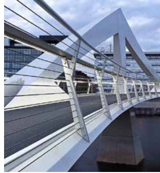
Image 10: Similar impression created by horizontal ropes used as guard rails by Jakob Rope Systems on a pedestrian bridge in England.
