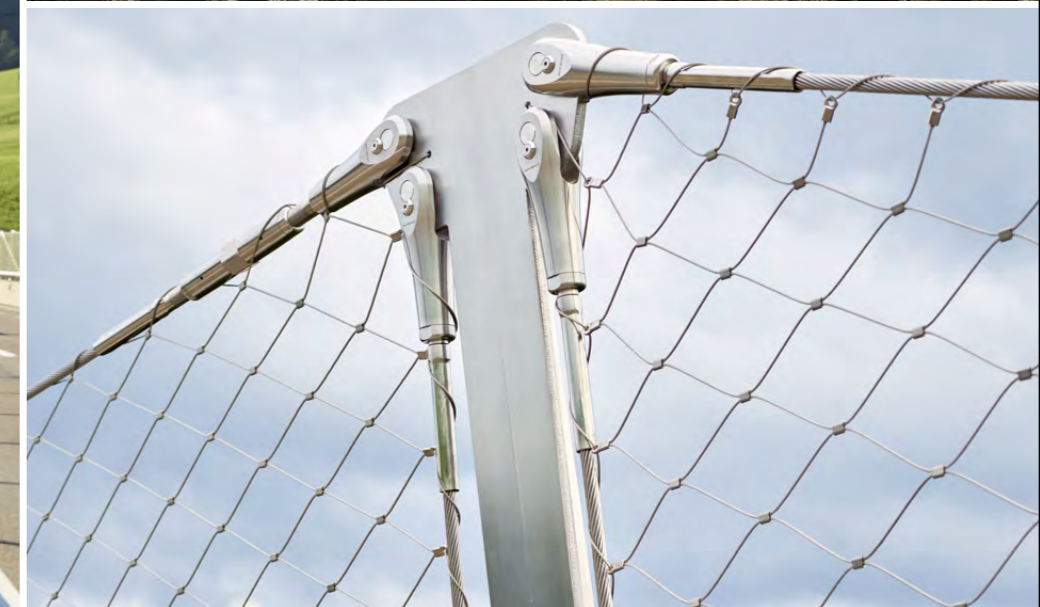
Hundwilertobelbrücke, Appenzell AR (CH)
